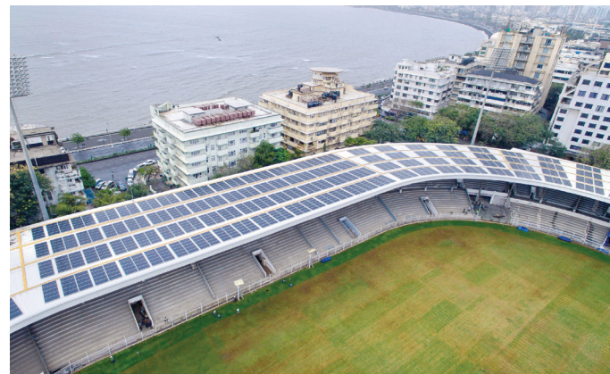
In 2018, Tata Power installed a solar rooftop plant on the stadium roof of the Brabourne Stadium. Known to be the world's largest installation on a cricket stadium, the plant generates 1.2 million units per annum
