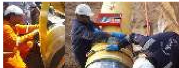
Permanent Composite Sleeve Repair - Clock Spring NRI
